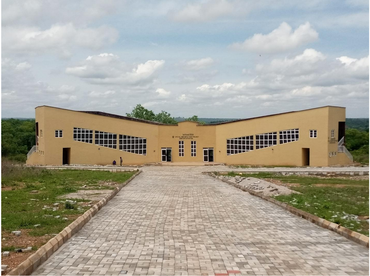
Tetfund 2018 High Impact Twin Lecture Hall
